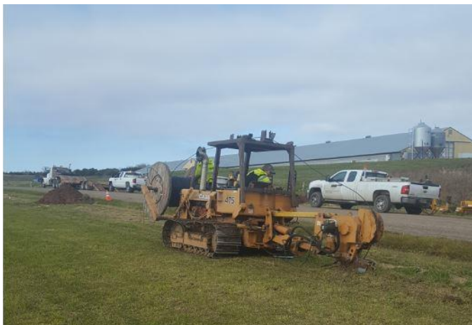
Fiber Line Installation
