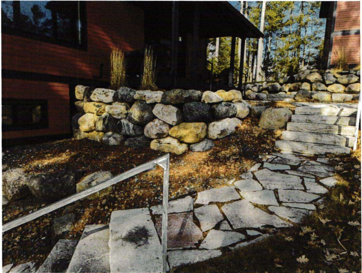
The rock landscaping (retainage) is necessary for the stability of the soils adjacent to the structure on this site which has significant slope toward the lake.
