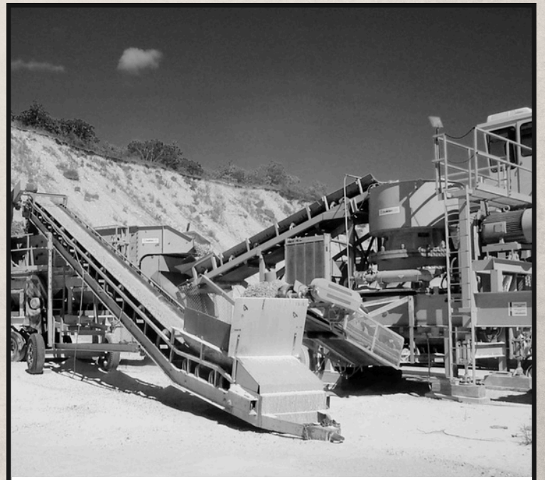
BARRON CO HWY DEPT CRUSHING OPERATION: 2003
