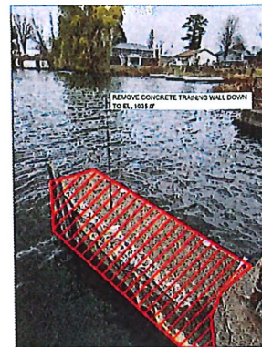
3. POWERHOUSE WASTEWATER GATE TRAINING WALL
