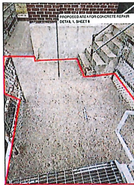
2. POWERHOUSE WALKWAY PLATFORM
