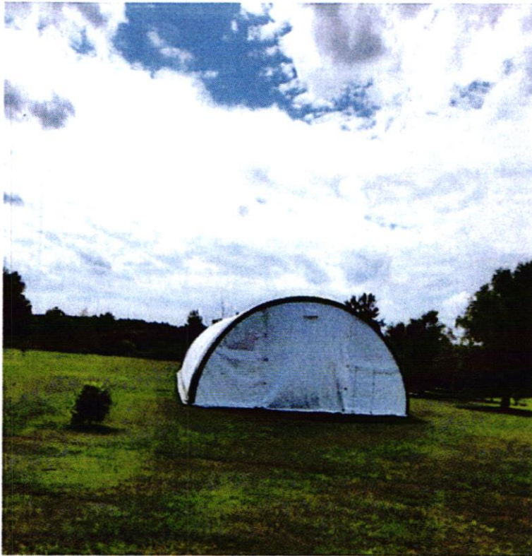
Accessory structure at 1382 24 3/8 Street
