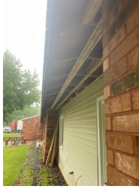
Almena soffit removed
